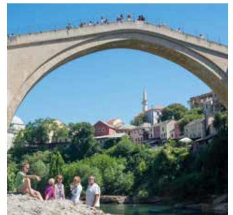
MOSTAR BRIDGE, BOSNIA & HERZEGOVINA
